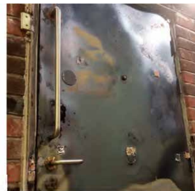
After Hose Stream Hardware still firmly attached
